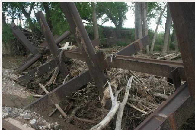
Vehicle barrier in the San Pedro riverbed clogged with debris. 2012. Scott Nicol.
