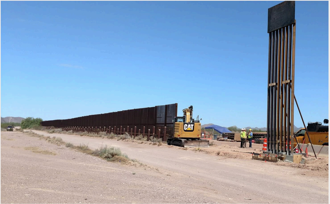
30-foot-tall bollard wall replacing 18 foot tall mesh border wall at Organ Pipe Cactus National Monument. 2019. Anonymous.
